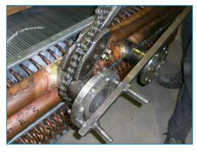
Installing screw-on flange
