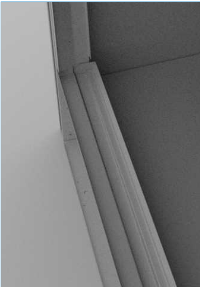
Water collection gutter
