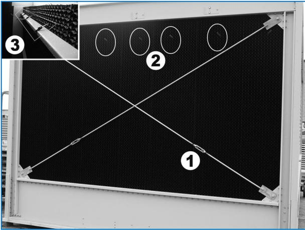
*Tie rod & straps for combined inlet shields*
