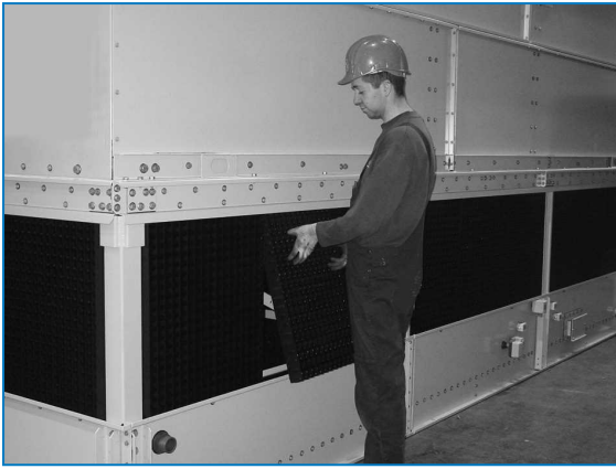
Remove combined inlet shields
