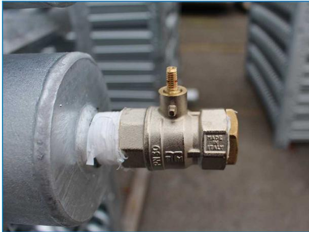
*Upper coil connection with pressure release valve on condensers.*
