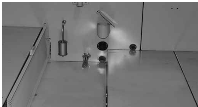
Figure 2: Cold Water Basin and Basin Strainer
