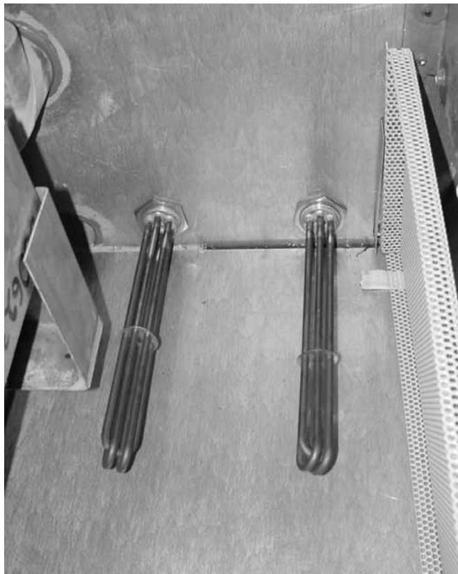
Figure 4: Sump Heaters
