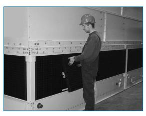
Remove combined inlet shields
