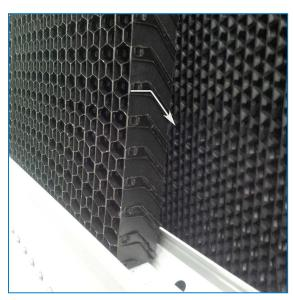
Orientation of the combined inlet shield
